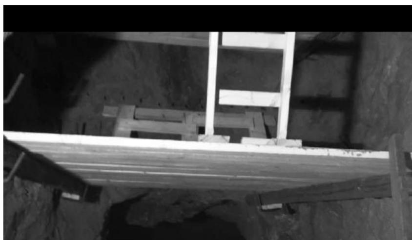
Picture no. 8 - Working platform in chimney
